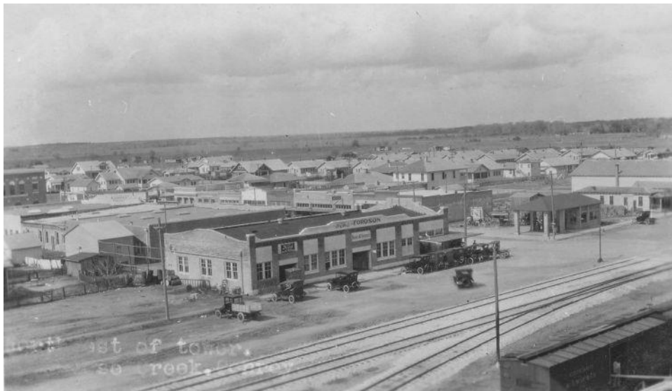
Image 10d. Henry Cathriner's Ford dealership is on the corner of Texas Avenue and Commerce Street. That building still stands. The Pruett garage is across the street and the Oiler Theater is barely visible on the far right.
