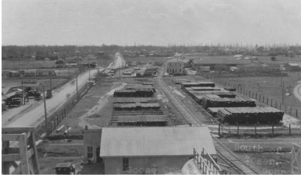
Image 10a. This series of five photographs was taken about 1923 from the concrete water tower located at the west end of East Pearce Street. This view is looking south down Main Street towards Pelly and the Goose Creek oil field. The large pipe lay-down yard was on property owned by Ross Sterling and further south was the Roberts McDonald Lumber Company. Courtesy of Denise Reineke Fischer.
