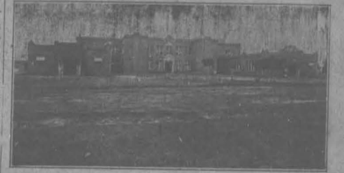
GRAMMAR SCHOOL BUILDING, GOOSE CREEK
